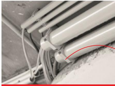
In conjunction with the UVB, the EC Euro-Clip fulfils the requirements of a closed clamp. This prevents the pipes from slipping out.
